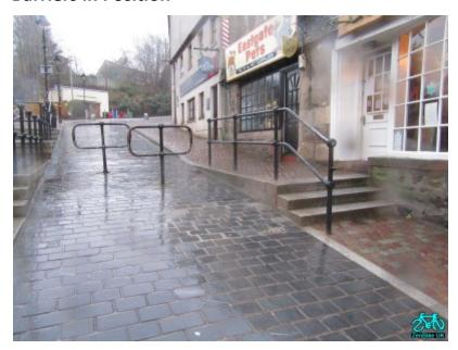
One footway was lost when it was replaced with stone cubicles used informally as alfresco extensions for the businesses opposite. A new, short flight of three steps was introduced into the footway in front of the businesses. The bollards were replaced by two offset, staggered barriers.
